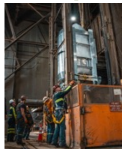
TPC moves underground Oct 2019
