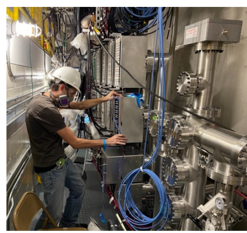
Electronics installation Fall 2020
